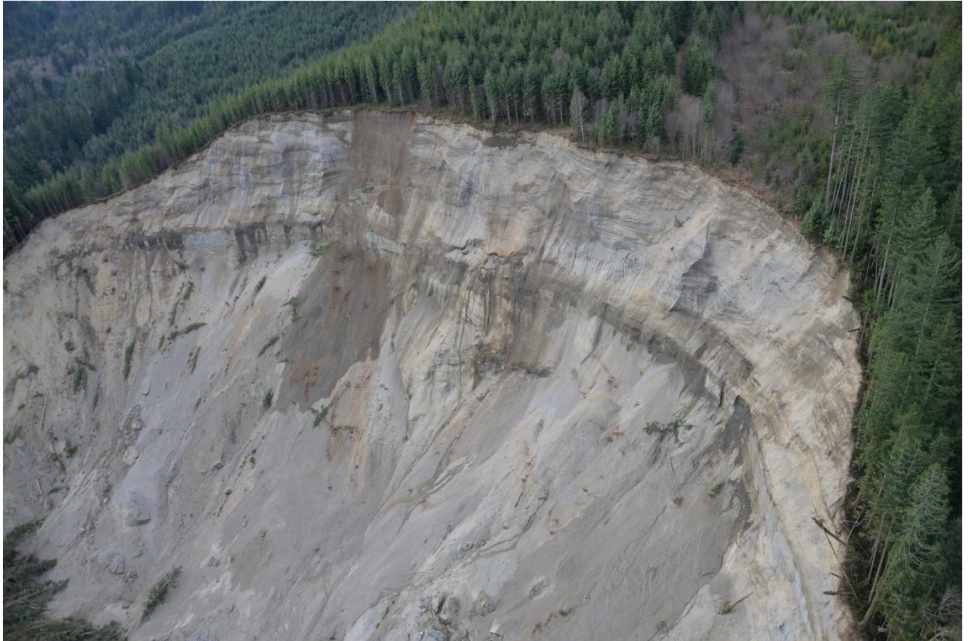
Caption: Landslide close up near Oso, Washington in 2014 (Source: Air Support Unit, King County Sheriff's Office)
