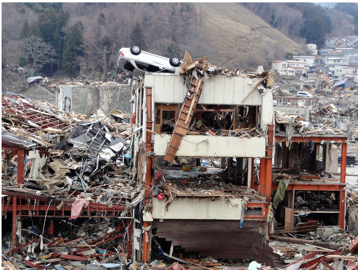
Caption: Damage from the 2011 Tohoku tsunami in Japan (source: NOAA NCEI).
