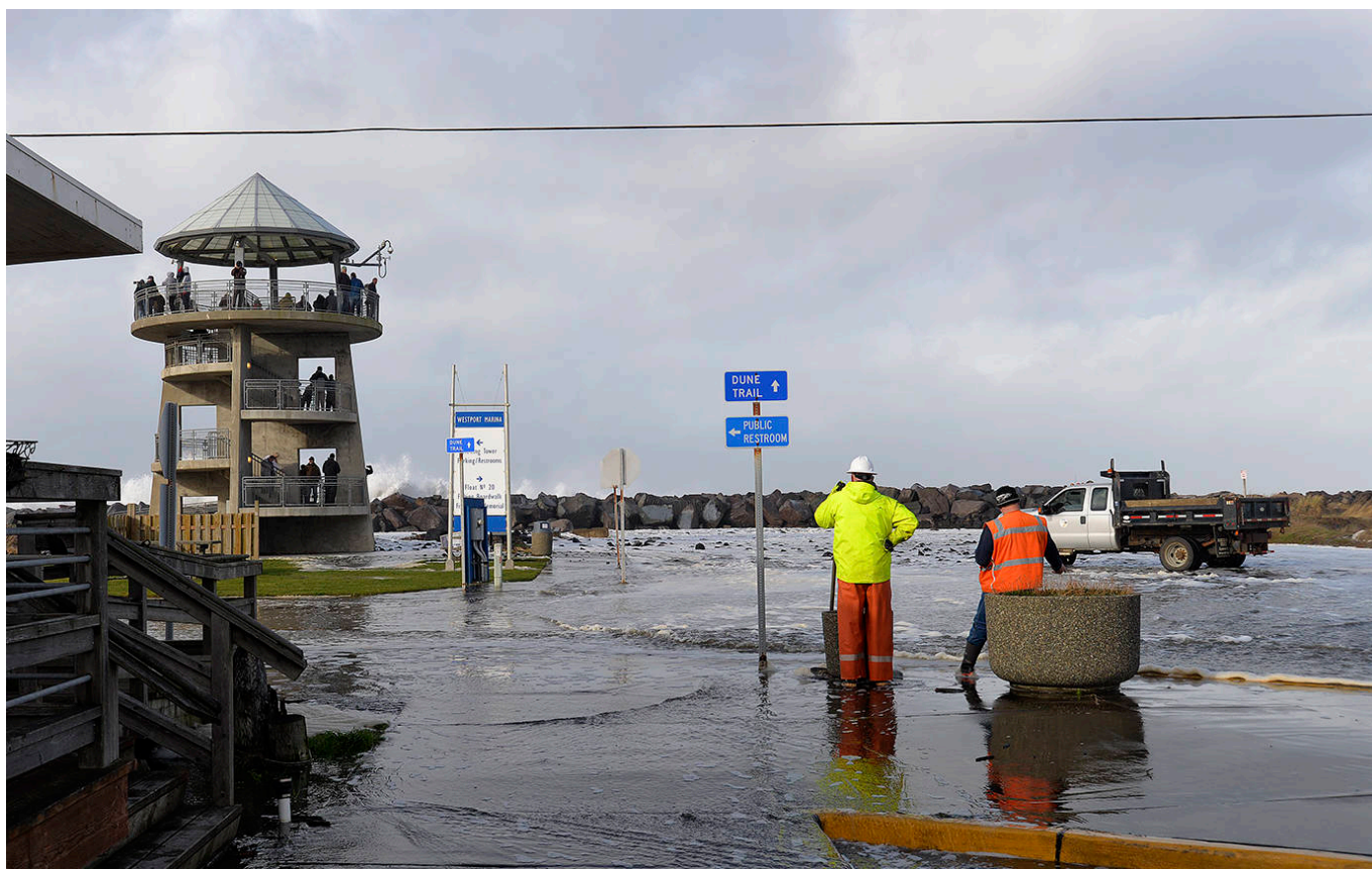
Caption: Waves pummeling the Westport jetty on January 18-19, 2018 caused flooding on several blocks of Westhaven Drive (source: Dan Hammock, The Daily World).
