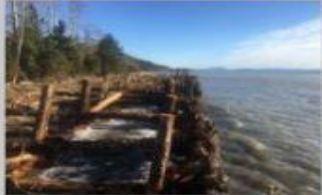
2 Chinook Shoreline Stabilization
