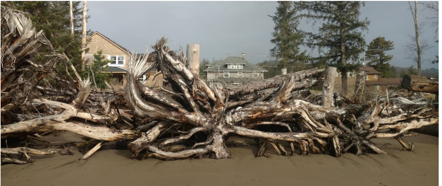
Root wads with intact trunks face the water, helping dissipate wave energy. (Photo credit: Jackson Blalock, The Nature Conservancy)
