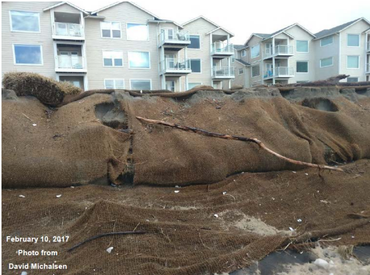
Figure 3-4: Ground-based photograph of emergency protection measures and coir mat on the seaward face of the erosion scarp representative of the condition in early February 2017 following an interval of winter storms
