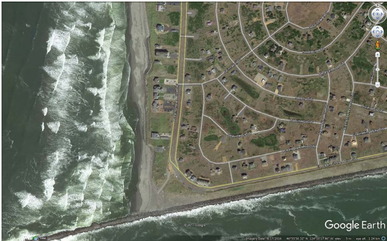
Figure 4-1: End effect erosion at the north and south end of rip-rap placements at Ocean Shores
