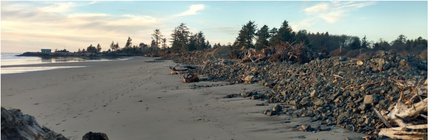
Cobble and woody debris move with waves, providing erosion control without increasing erosion along adjacent shorelines. (Photo credit: Jackson Blalock, The Nature Conservancy)
