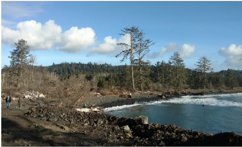
Constructed cobble feeder bluff (in foreground) feeds beaches (in background) with protective material (left). (Left photo credit: Jackson Blalock, The Nature Conservancy; right image credit: Pacific Conservation District)
