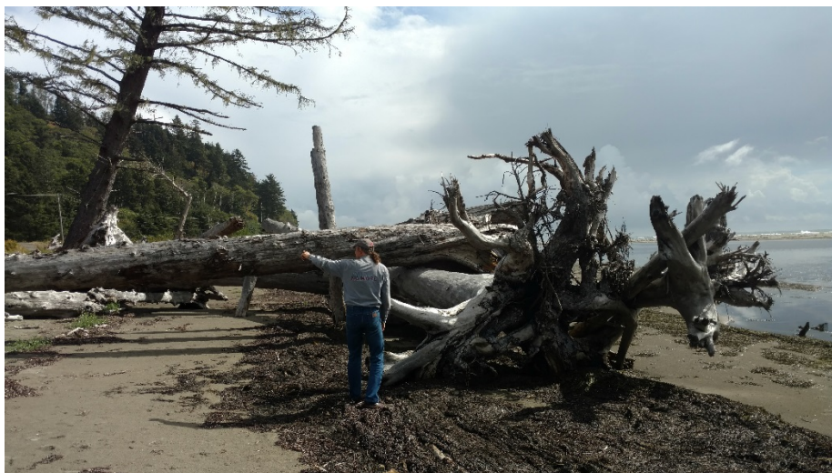
David Cottrell of Washaway No More shows how large wood structures have been anchored into banks and other wood. Placing large wood structures at intervals effectively disrupts the longshore current and helps retain sand, preventing further erosion. (Photo credit: Jackson Blalock, The Nature Conservancy)
