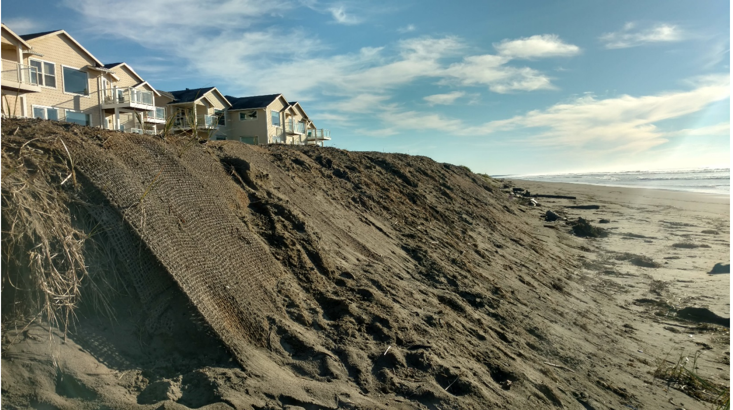
After years of back-and-forth erosion and emergency repairs, Westport by the Sea’s artificial dune is covered with sand (some mechanically deposited, some deposited by wind). Note exposed coir matting (right). (Photot credit: Jackson Blalock, The Nature Conservancy)
