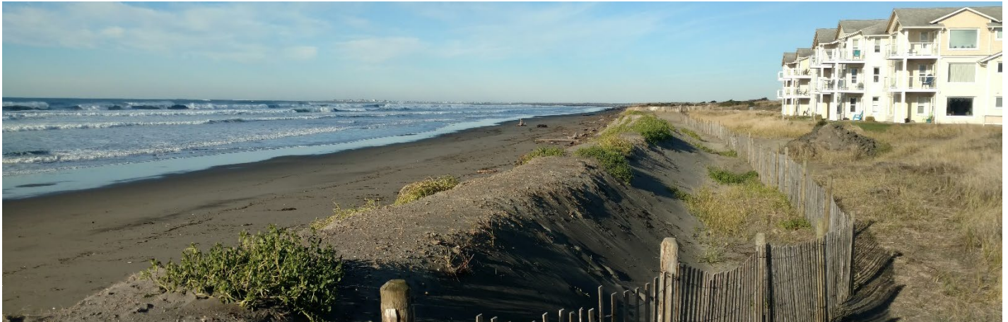
An artificial dune defends against erosion while sand fencing collects wind-blown sediment. (Photo credit: Jackson Blalock, The Nature Conservancy)
