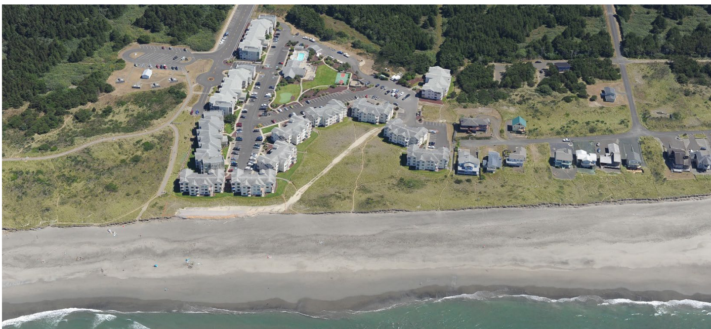
Access route for repairs and continued erosion management is visible as a sandy line between the parking lot and artificial dune. This road has been relocated, but remains in use for adaptation activity. (Photo credit: Washington State Department of Ecology's Coastal Atlas)
