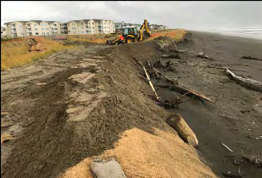
Buildup and extension of dike
