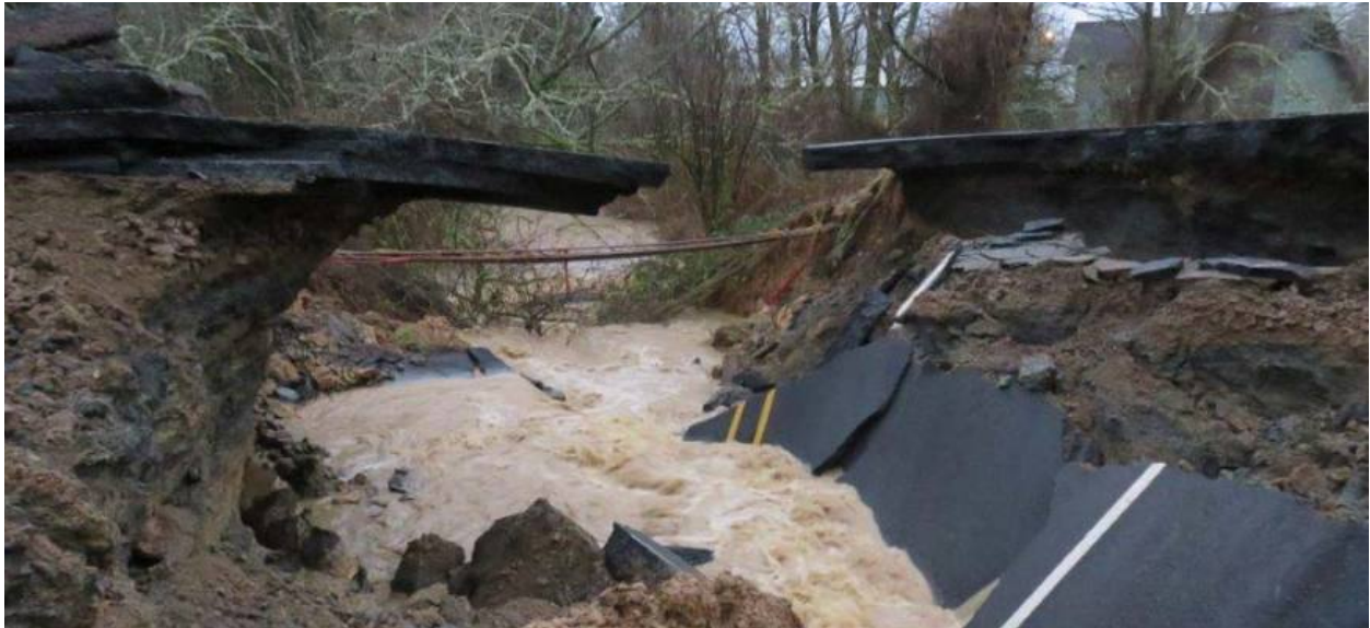
SR 4 west of Naselle is closed between US 101 & SR 401 due to a collapsed culvert (source: mynorthwest.com).
