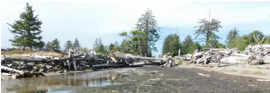
Strategically-placed woody debris protects the drainage canal and Highway 105 in North Cove, WA from high waters (source: Molly Bogeberg, The Nature Conservancy)
