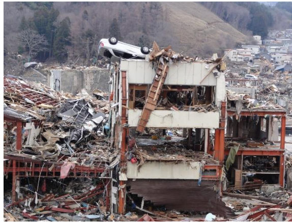
Damage from the 2011 Tohoku tsunami in Japan.
