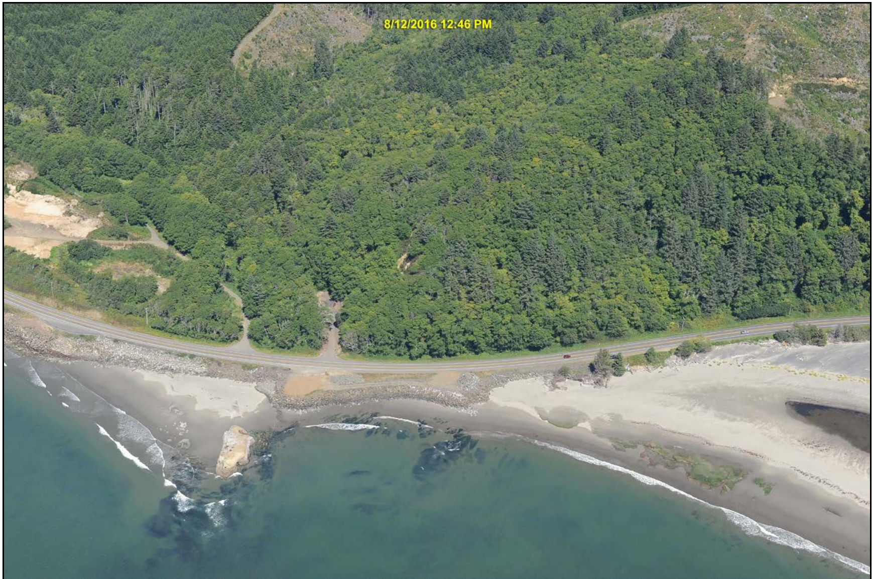
Figure 27. Cape Shoalwater – Land connection of Graveyard Spit (note shoreline protection and rock outcroppings)
