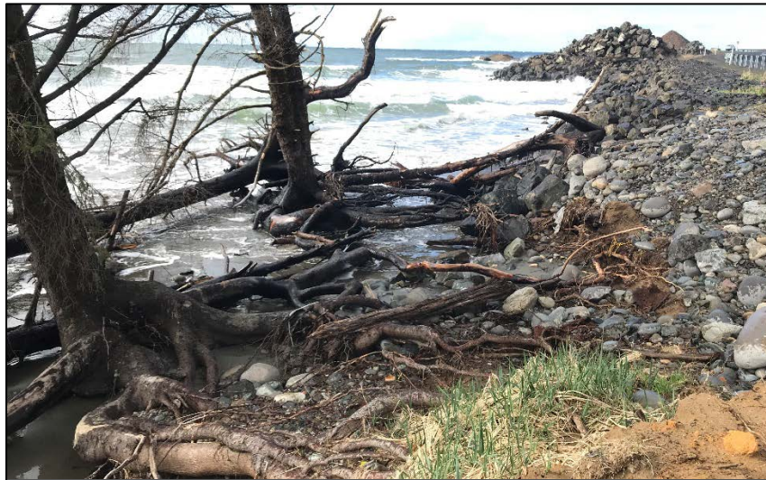
Figure 8 Loss of remnant terrace material at the west end of the project after the January storms
