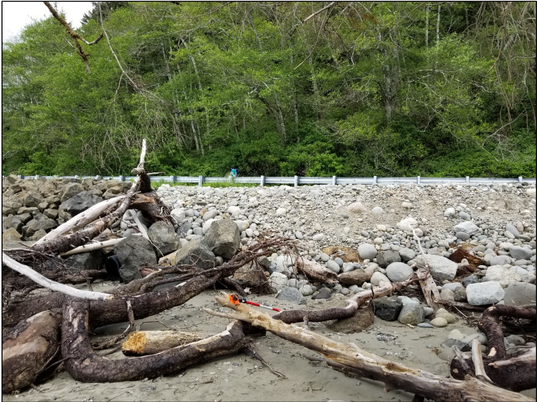
Figure 11 Photo of slumping material in the west transition area
