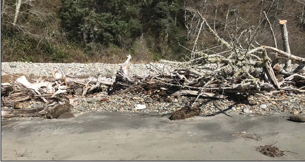
Figure 12 Photo of gravel transported east from the eroded segment of the dynamic revetment
