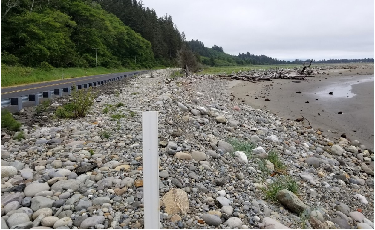
Figure 11. Photo from Section 1 of cobbles transported eastward along the toe of the dynamic revetment.
