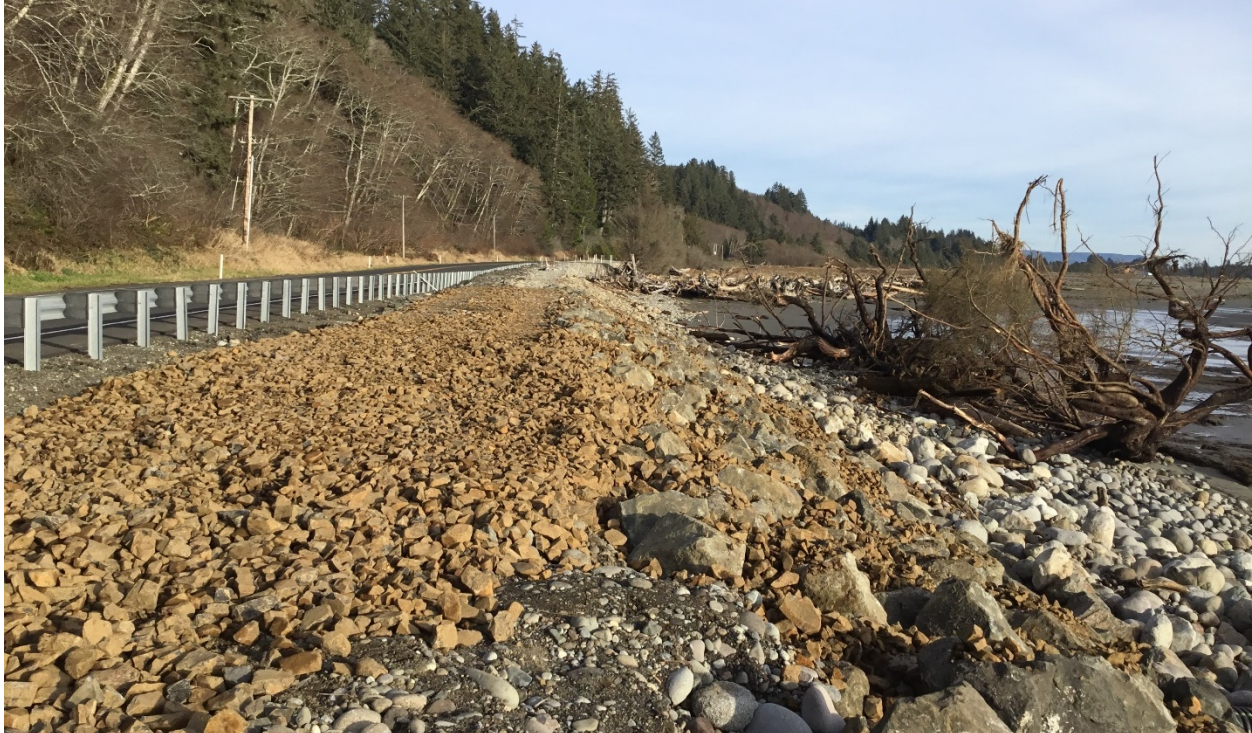
Figure 9. Photo of the completed January 2019 riprap repair.
