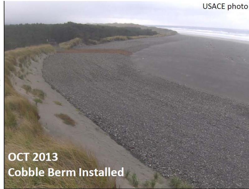
South Jetty Dynamic Revetment
