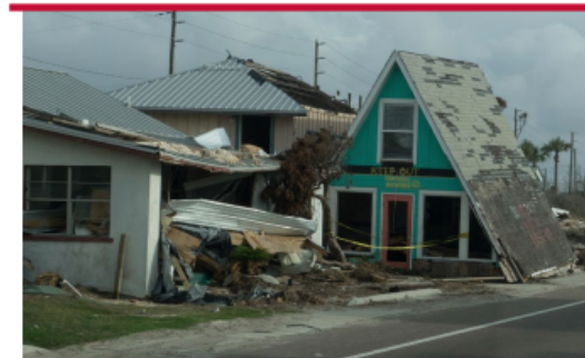
Damage caused by Hurricane Michael in Mexico Beach, FL Source: Shutterstock
