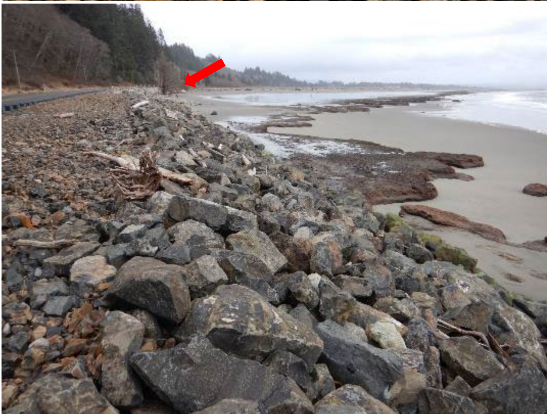
Figure 2-13. Eastern end of pilot dynamic revetment; above, February 2019; below, February 2021. Note red arrow indicating the same tree in both photos. Additional rock in foreground was placed in December 2020.
