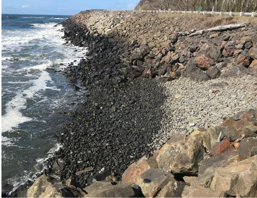
Figure 5-11 Partial rounding of angular cobble placed as part of rock revetment, just west of Graveyard Spit.
