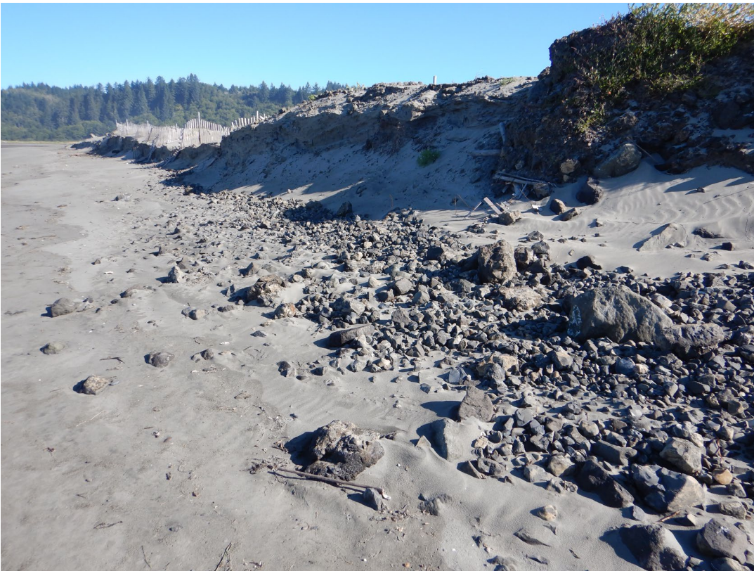
Figure 2-9. Aeolian and wave erosion of angular rock and dune sand, Empire Spit Dune restoration project. Above: looking directly at dune. Below: looking north along toe of dune.
