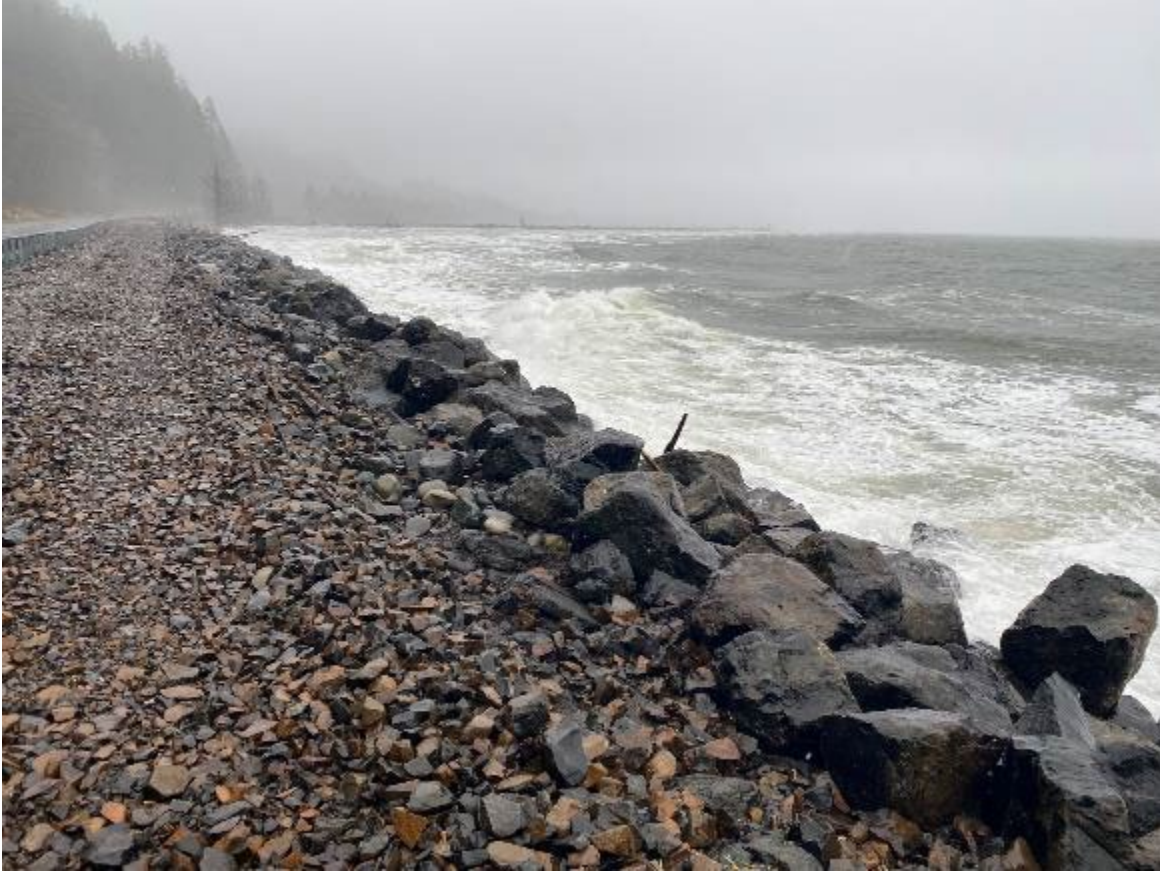
Figure 5-8. Location of western transition, during February 28, 2022 storm.
