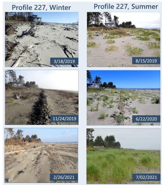
Figure 6. This photo series shows sand accumulation and vegetation establishment between 2018 and spring of 2021 on a selected monitoring profile (profile 227) of the North Cove Dynamic Revetment Project. Provided by Hannah Drummond / CMAP.
