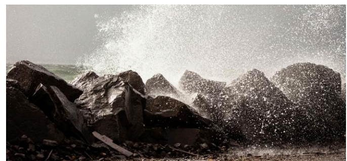
Debris-filled waves crash over the US 101 seawall in Chinook (Natalie St. John, Chinook Observer)
