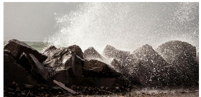
Debris-filled waves crash over the US 101 seawall in Chinook (Natalie St. John, Chinook Observer)
