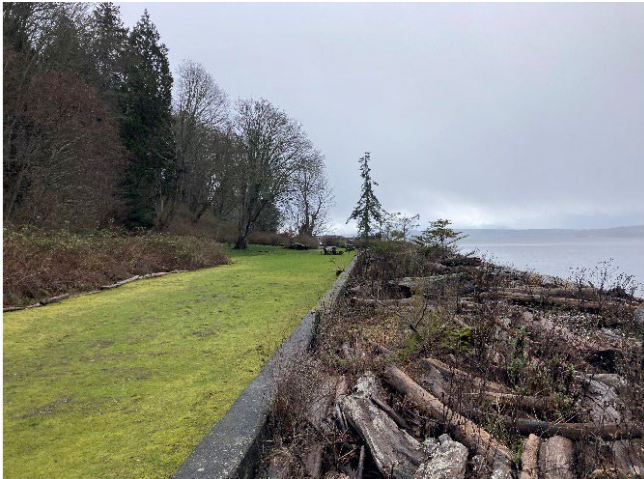
The northern part of Cama Beach State Parks receives the sediments and logs transported in the drift cell. The beach would move landward by building upwards but is impeded by armor.
