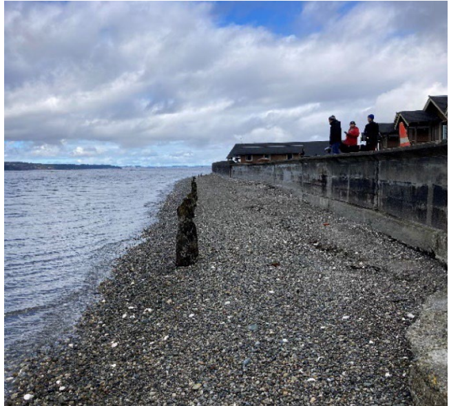
Shoreline armor at Cama Beach State Park is trying to protect the cabins by preventing bank erosion. As longshore currents try to move beach sediment northwards, the beach and foreshore narrow.
