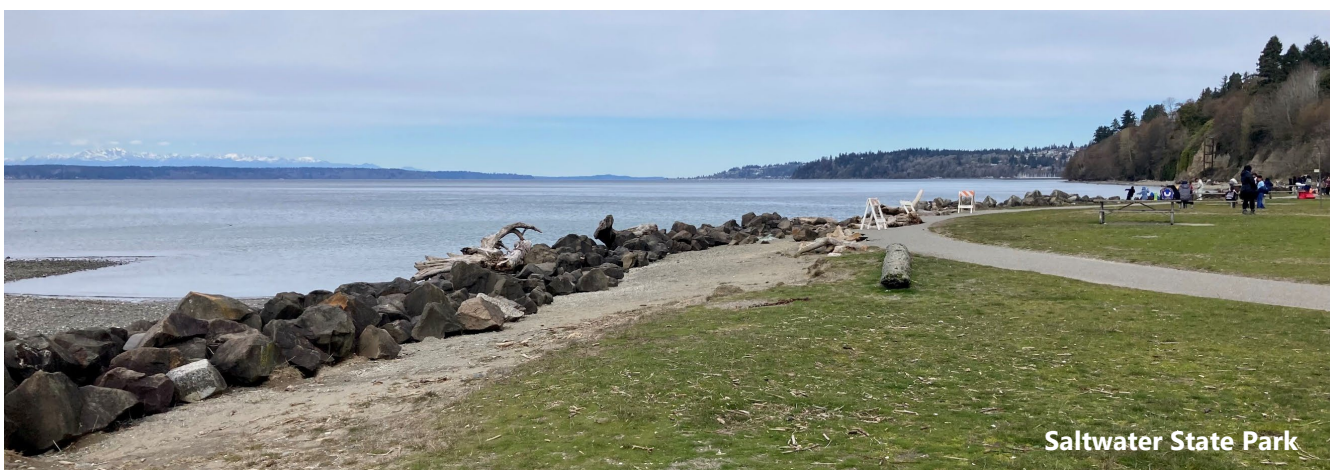
Figure 33. Shoreline Armor at Saltwater State Park Is in the Planning and Design Process To Be Removed and Restored.
